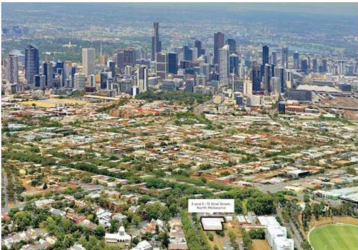
Fridcorp's North Melbourne development site
